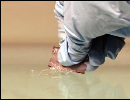
Remove Excess Resin
